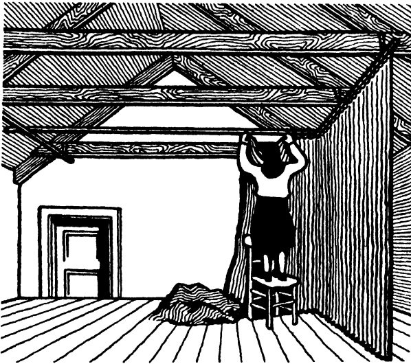
Fig. 5. Fit-up using Existing Features of Roof for Support.
