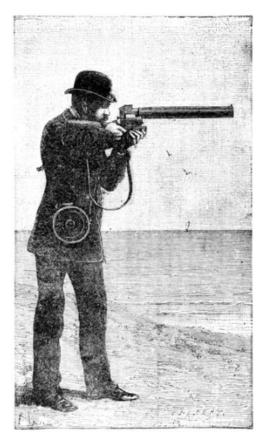
FIG. 17.—MODE OF USING THE PHOTOGRAPHIC GUN.
