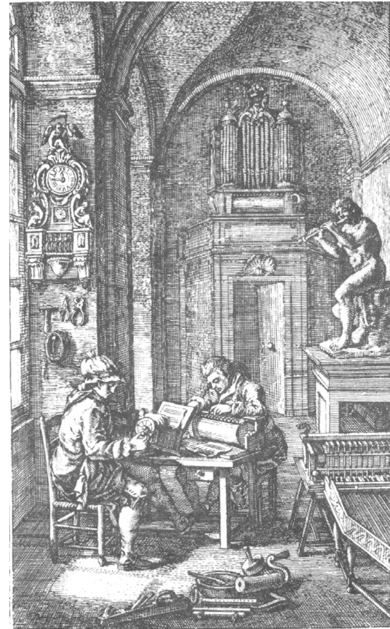
Figure 6.22 Frontispiece from Father Joseph Engramelle’s Tonotechnics , 1775. Around the room are several automated musical instruments powered by clockwork: a pipe organ over the door, a clock with a carillon in the window, a self-playing harpsichord and a mechanical flute player.
