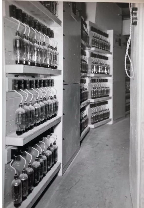
Figure 5. Console and dimmer racks at Reykjavik (Strand Archive 1950; Theobald 1950)
