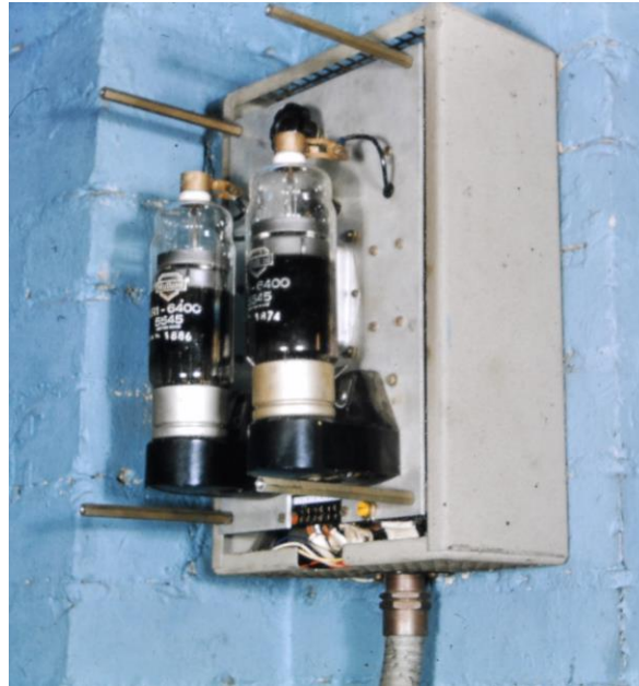
Figure 45. Brown Boveri Thyralux dimmer (cover removed) (c1952a)
