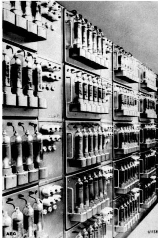
Figure 48. AEG ‘Regolux’ thyatron dimmer racks (three dimmers per panel), Germany, 1954 (Frank 2015)
