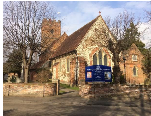
Figure 64. Littleton Parish Church
